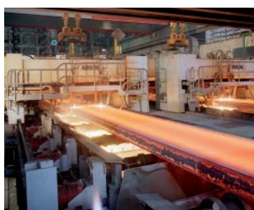
Twin-stand slab casting machine
